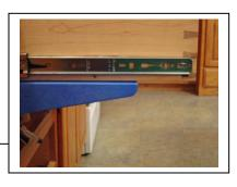
For frameless cabinets, reverse the brackets end for end and swap sides so the long toe points inward as shown. Move the brackets into position so that they contact the base of the slides. Clamp into place as shown and continue mounting the drawer box as described in the framed cabinet example above,
